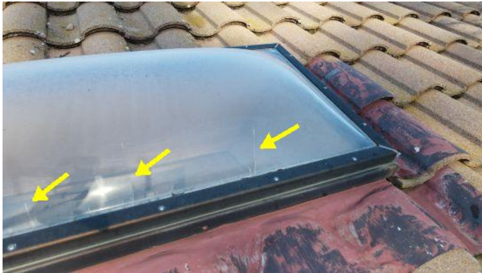
Example of cracks in skylight lense
