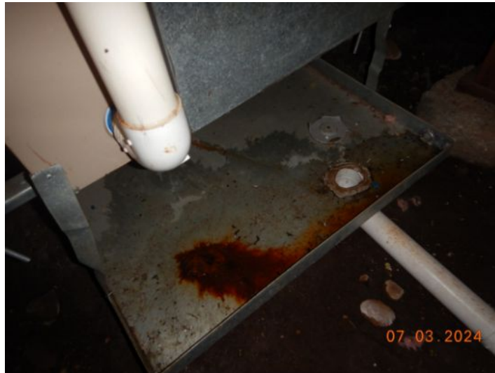
Rust and moisture in drip pan
