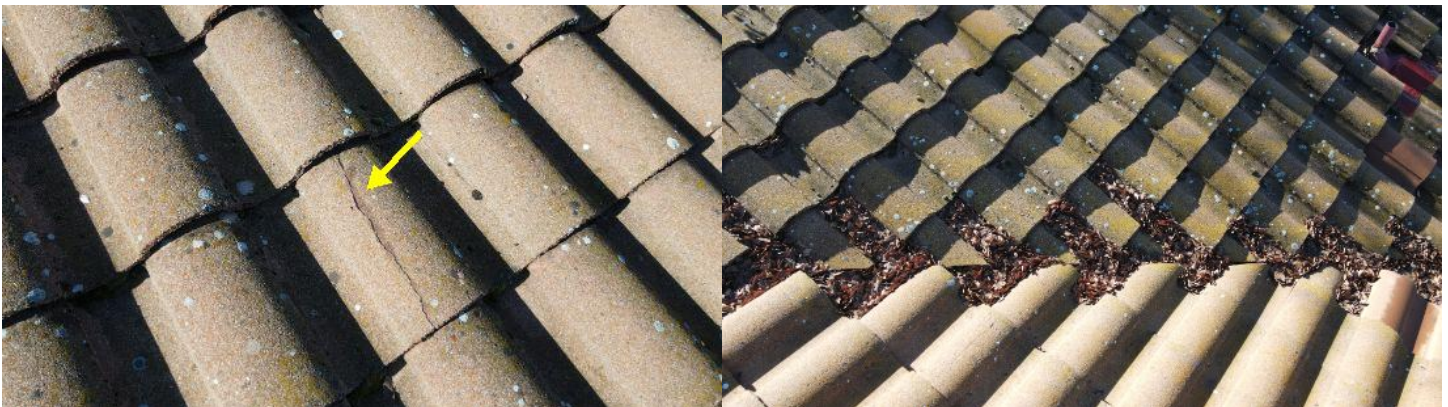
Example of cracks in tiles
