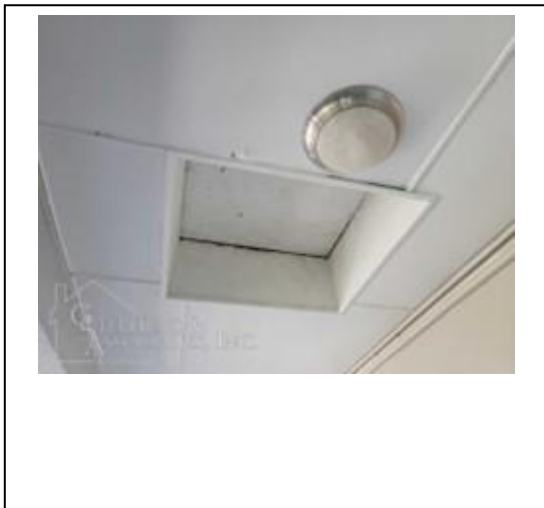
Roof Access Hatch
