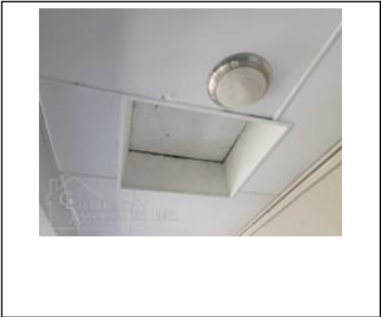
Roof Access Hatch
