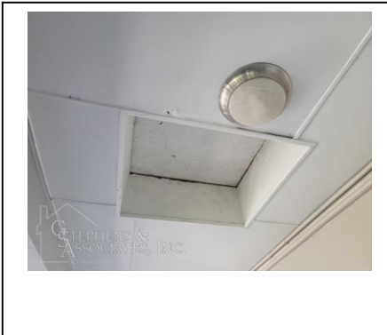
Roof Access Hatch
