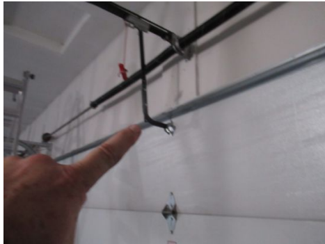
no reinforcing bracket for arm extension
