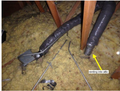
bathroom duct laying on attic floor
