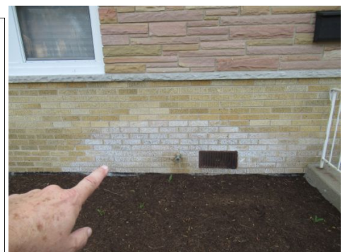
Efflorescence
