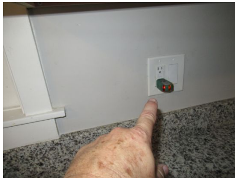
receptacle&gt;reversed polarity
