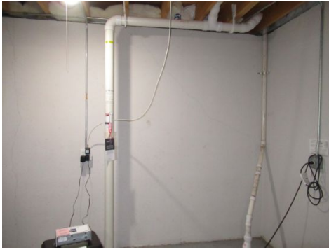
active radon mitigation pipe
