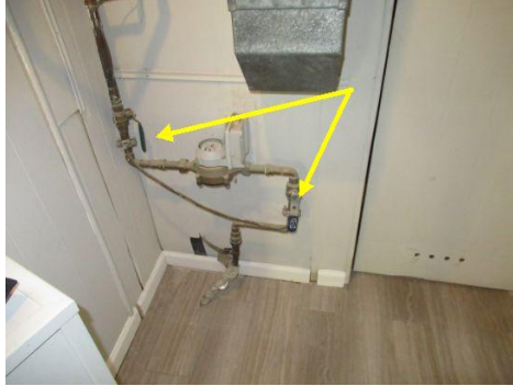
main water shut off valve / meter
