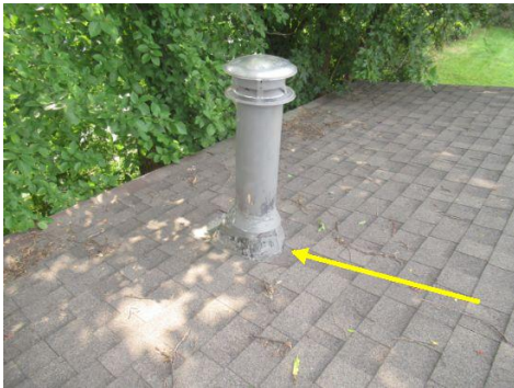
flashing&gt;vent
