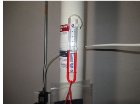
manometer for radon mitigation system
