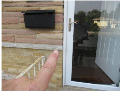
flashing/caulk not finished
