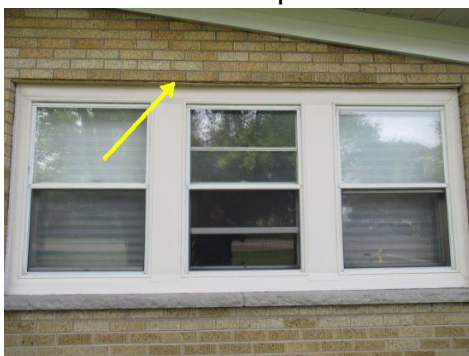
lintel above window>rusted
