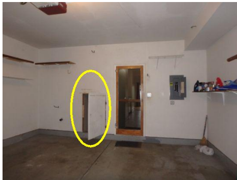
breach in the fire separation wall
