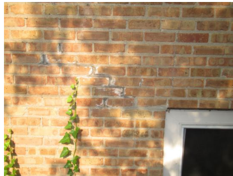
mortar repairs
