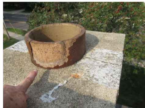
liner damage / no rain cap
