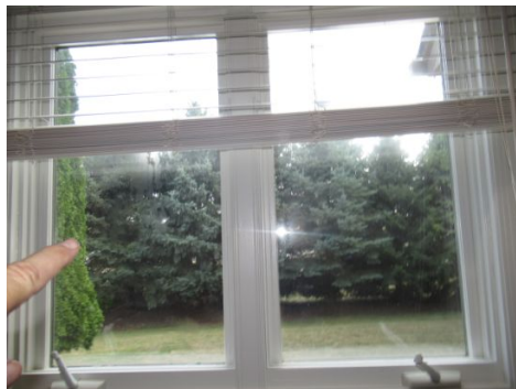
condensation between glass panels
