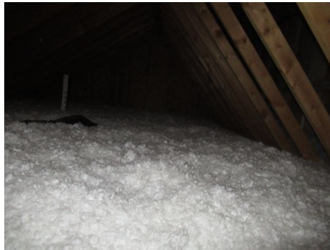
example of attic insulation
