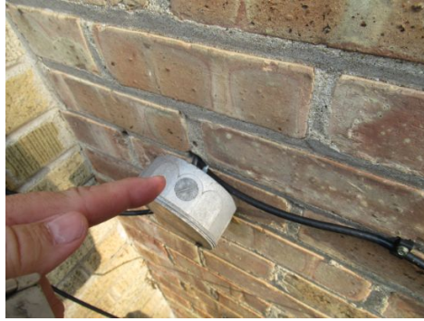
loose junction box/exposed wiring
