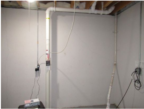
active radon mitigation pipe
