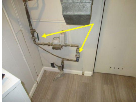
main water shut off valve / meter
