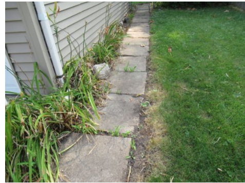
walkway>uneven walking surface
