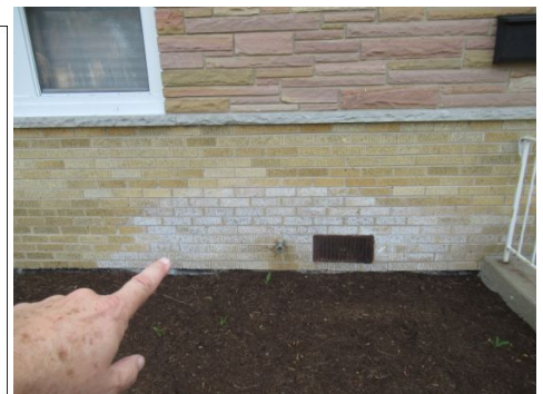
Efflorescence
