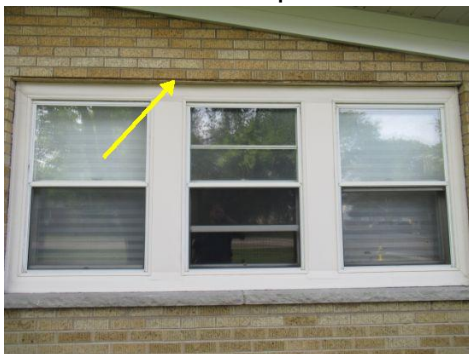
lintel above window &gt; rusted
