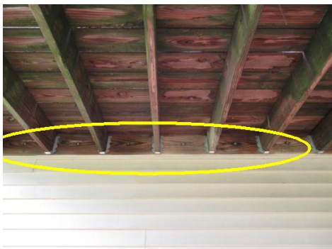
ledger board flashing not found / improper bolt pattern
