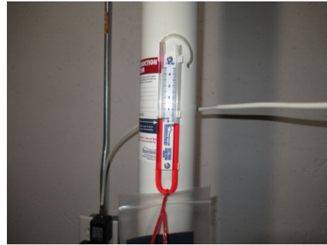
manometer for radon mitigation system
