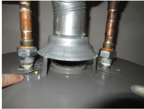
melted escutcheon rings
