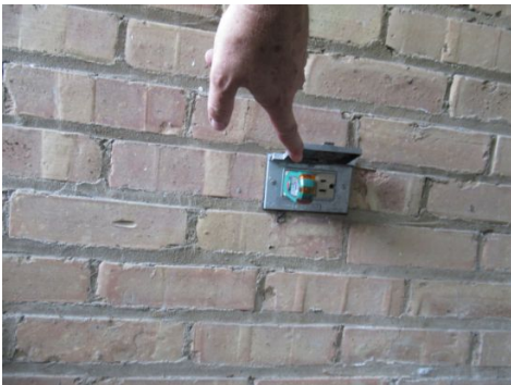
Receptacle did not respond to GFCI testing
